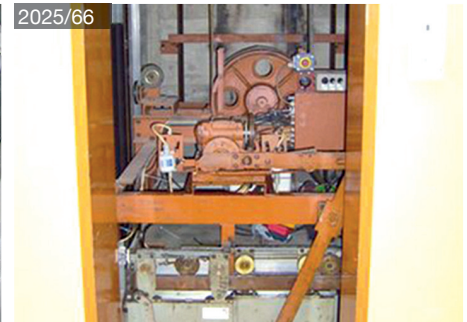
Haushahn TS54 telescope
