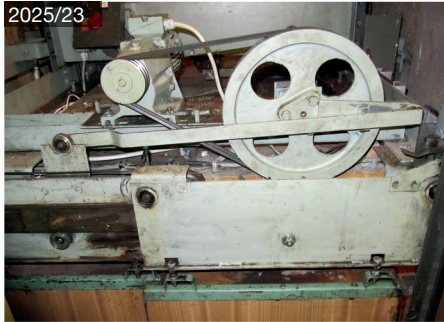
DOVER HD telescope 2025/26
