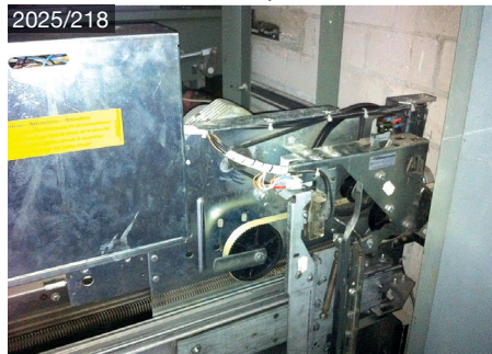
Schindler QKS11 telescope
