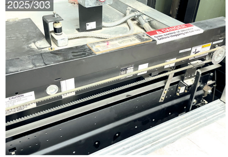
UNITEC AT400 Door Operator
