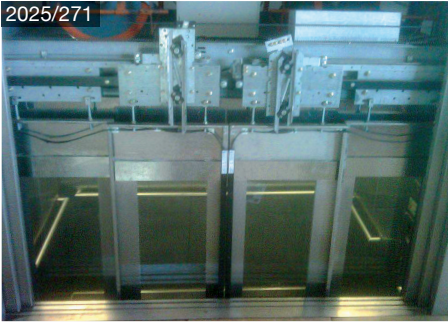
Thyssen D6C Prisma telescope 2025/274
